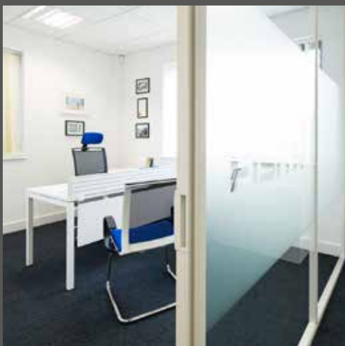
Office separated from the main office area by full height glazed partitioning with FISITA logo
