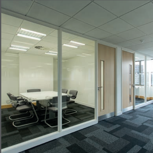
Solid and glass partitioning was used along with full-height maple doors to create meeting spaces
