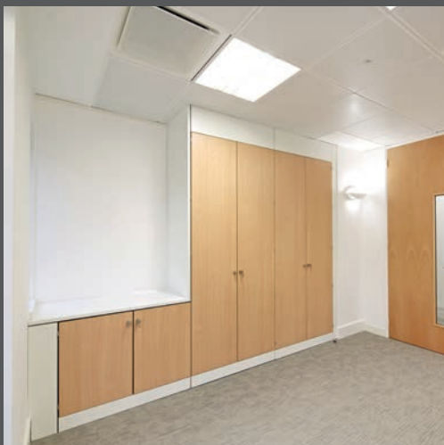
Fitted StorageWalls were installed to provide a neat storage solution
