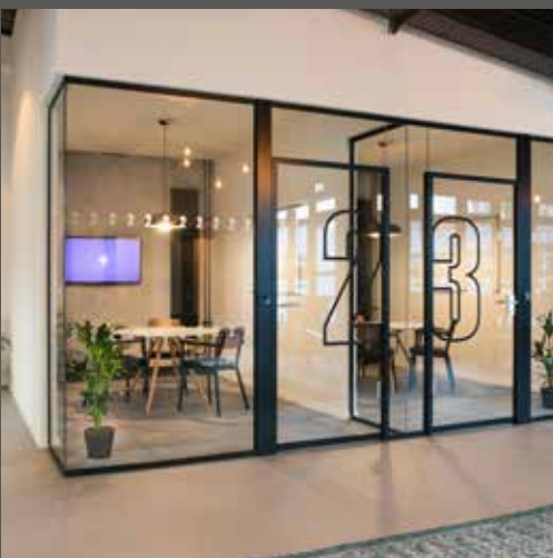
Meeting room with glass partitioning and manifestation.
